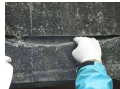
④ 補修材充填
